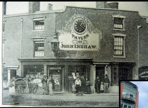
The Steam Clock Morville St at Sherborne St
